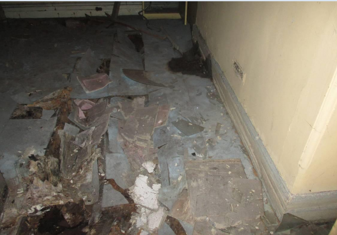
Floor tiles in building 1. No ACM's detected
