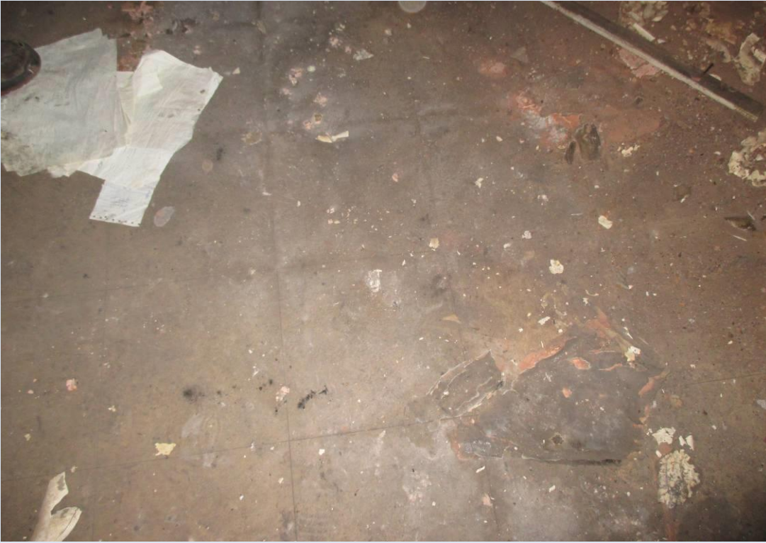
Floor tiles in building 1. No ACM's (asbestos containing materials) detected
