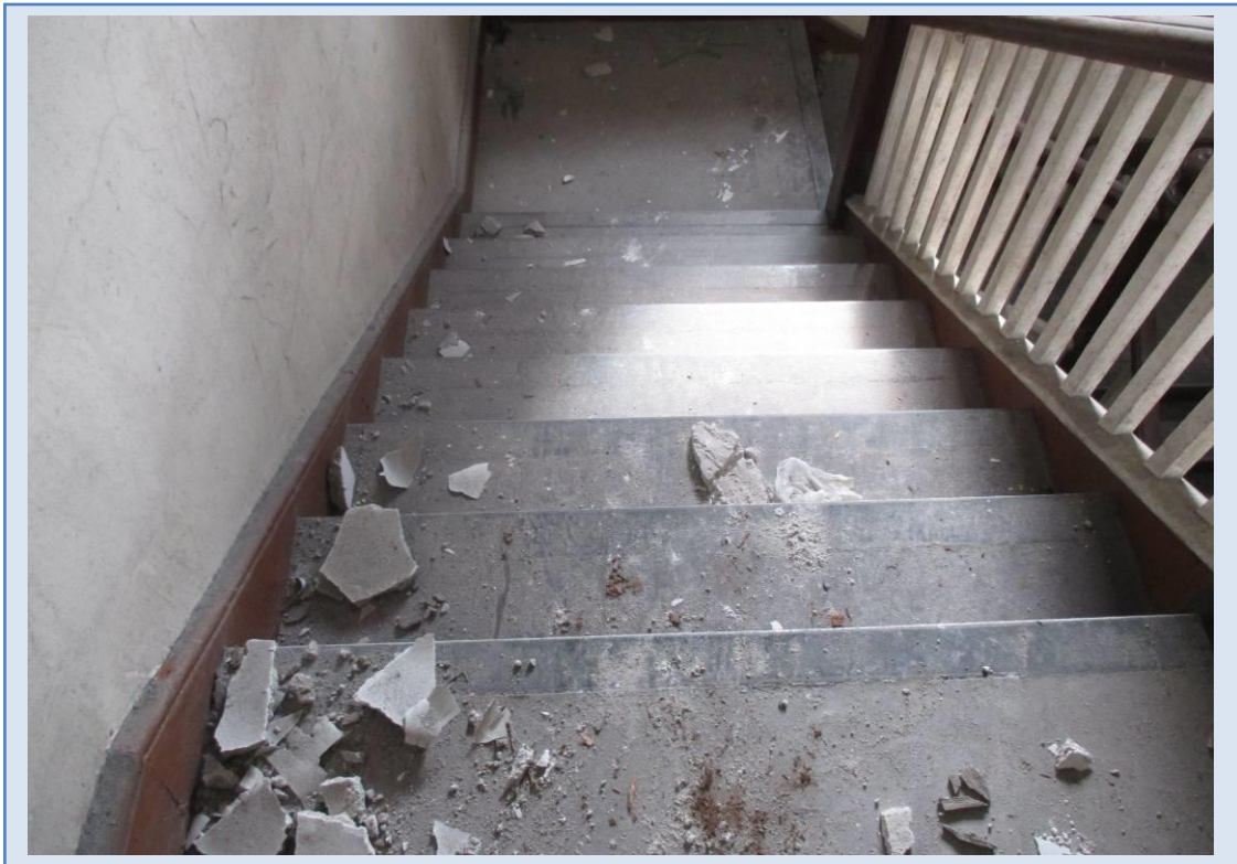
Stair nosing in building 4. No ACM's detected
