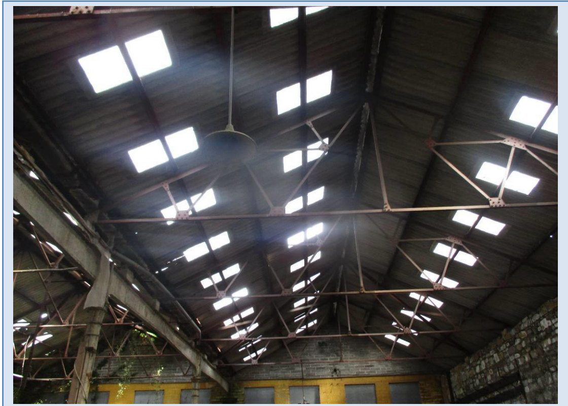
Asbestos cement roof sheeting in Building 7
