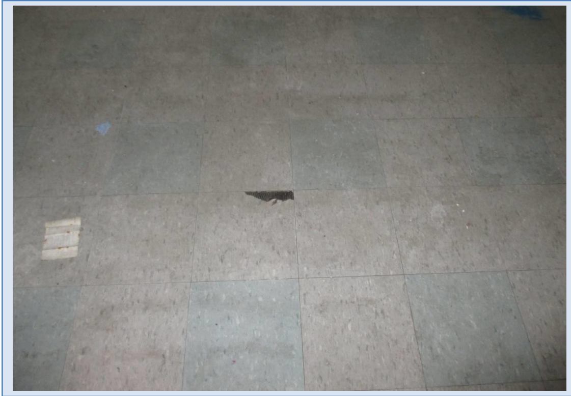
Floor tiles in building 5. No ACM's detected
